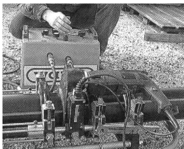
Sanfrenarea capetelor si aducerea lor in plan paralel
